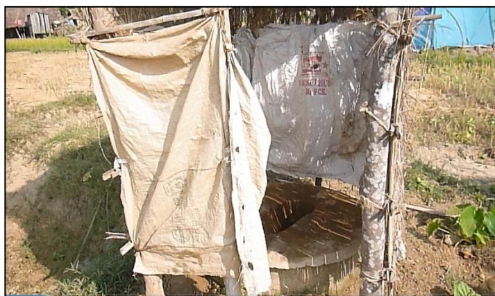
A simple pit latrine with slab at Baniyabar, Bardiya
